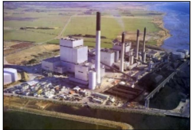
Figure 6b: ALSTOM Power Elsam project in Denmark (Nordjyllandsværket #3) (Net Ouptut: 385 MW, Efficiency (LHV): 47%)
