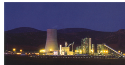
Puertollano IGCC Power Plant
