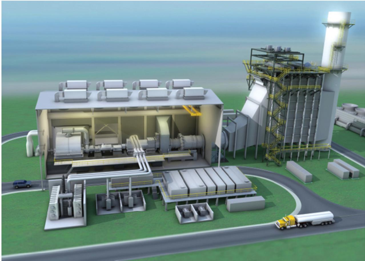
**1. Model of efficiency.** GE launched its FlexEfficiency 50 Combined Cycle Power Plant in May—a 510-MW power plant capable of offering a fuel efficiency of 61% and more. *Courtesy: GE*
