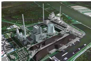
The 912 MW RDK 8 plant will be one of the first hard coal fired power plants in the world to run on steam at 600 °C to 620 °C
