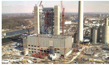
The steam generator operates on the once-through forced-flow operating mode, designed for ultra-supercritical steam parameters
