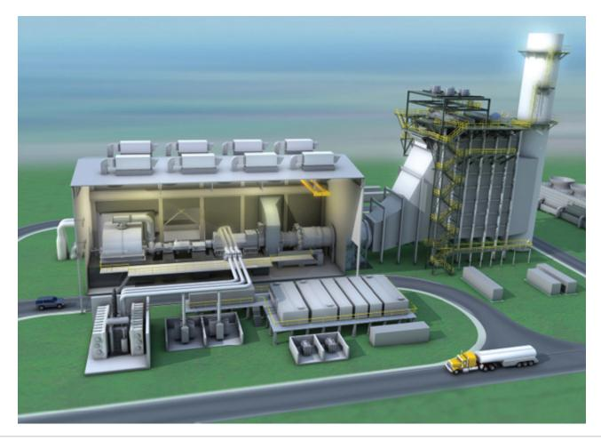
**1. Model of efficiency.** GE launched its FlexEfficiency 50 Combined Cycle Power Plant in May—a 510-MW power plant capable of offering a fuel efficiency of 61% and more. *Courtesy: GE*
