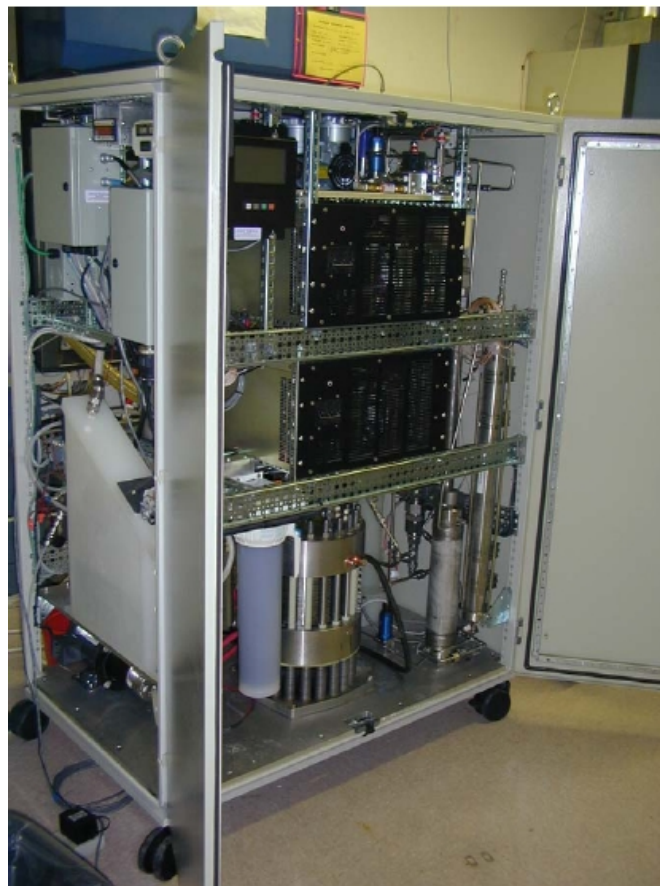
PEM high pressure electrolyzer system
