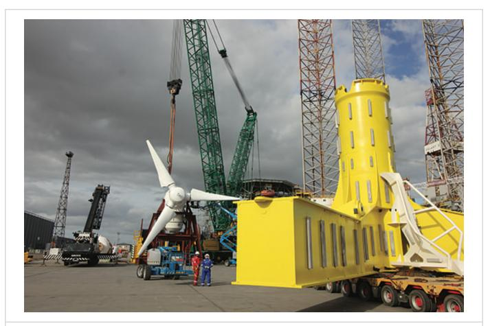
**1. Ocean energy.** The MeyGen Phase 1A array has four 1.5-MW tidal stream turbines—three, like the one shown here, supplied by ANDRITZ HYDRO Hammerfest and one supplied by Atlantis Resources. *Courtesy: ANDRITZ HYDRO Hammerfest*
