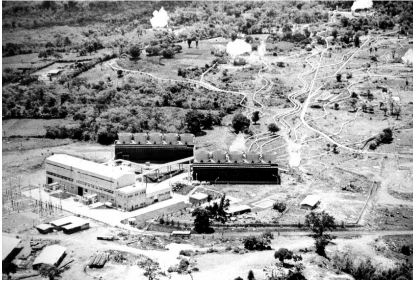
Figure 8.2 Ahuachapan geothermal facility after commissioning around 1977 (DiPippo, 1978).
