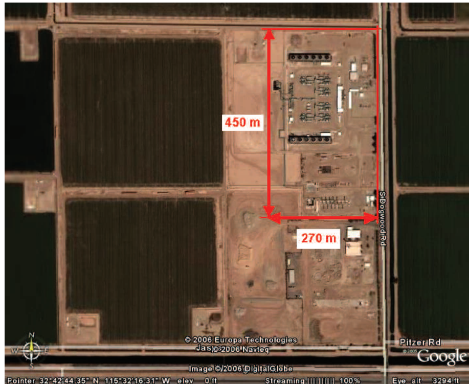
Figure 8.4 Aerial view of the SIGC binary plant near Heber, Calif. (Google Earth, 2006).
