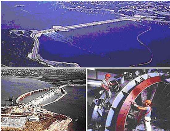
• Fig. 5. The La Rance tidal power station in France [13].
