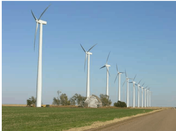
Figure 21. Representative Wind Farm: Gray County Wind Farm (Kansas)
