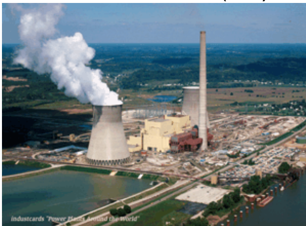
Figure 11. Representative Pulverized Coal Plant: Gavin Plant (Ohio)
