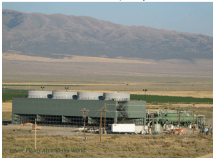
Figure 24. Representative Geothermal Plant: Raft River Plant (Idaho)
