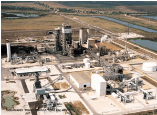
Figure 14. Representative IGCC Plant: Polk Plant (Florida)
